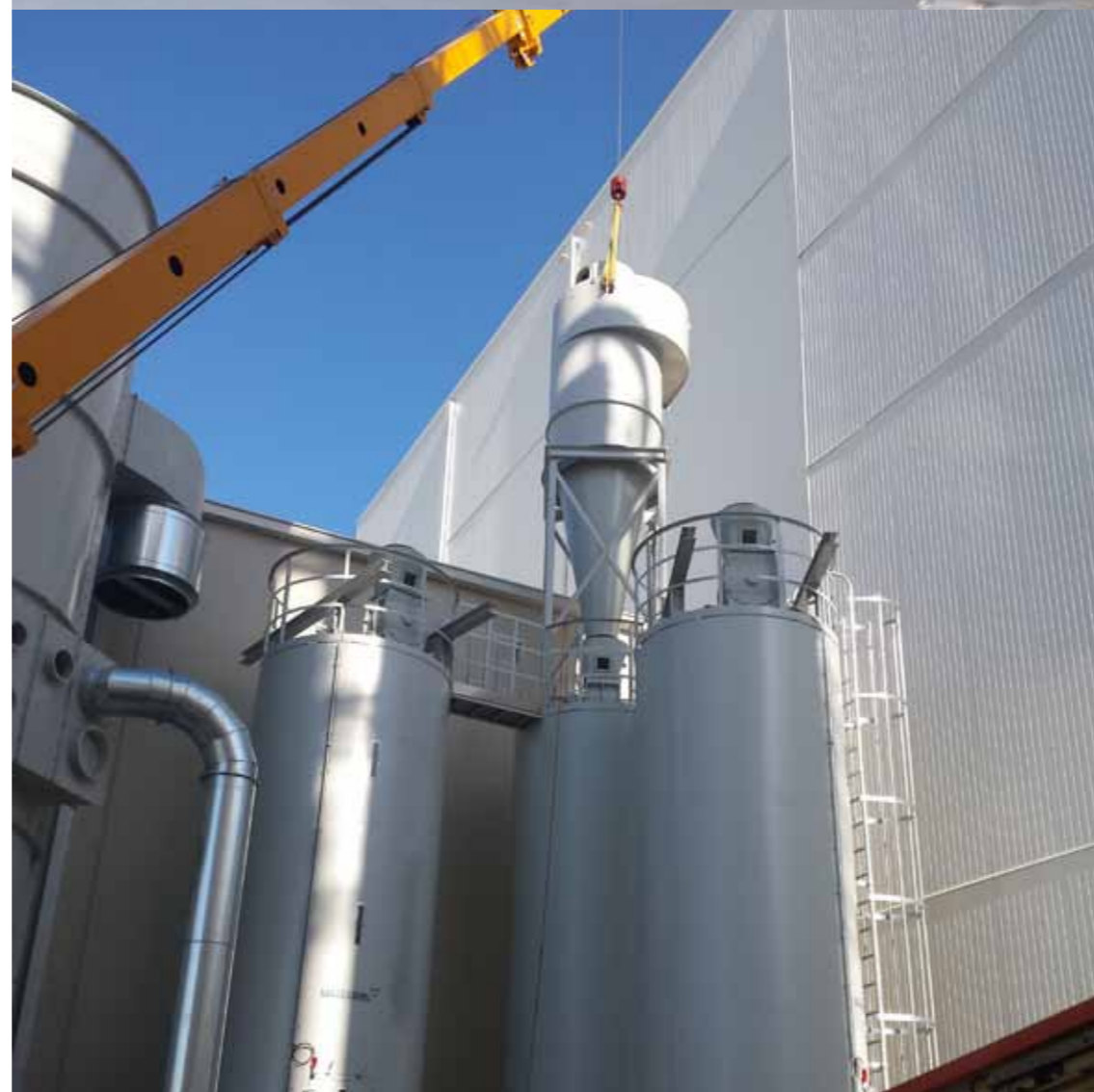
DUST COLLECTOR SYSTEMS FOR THE RECYCLING OF SANDING DUST WITH STORAGE IN BIG BAGS
