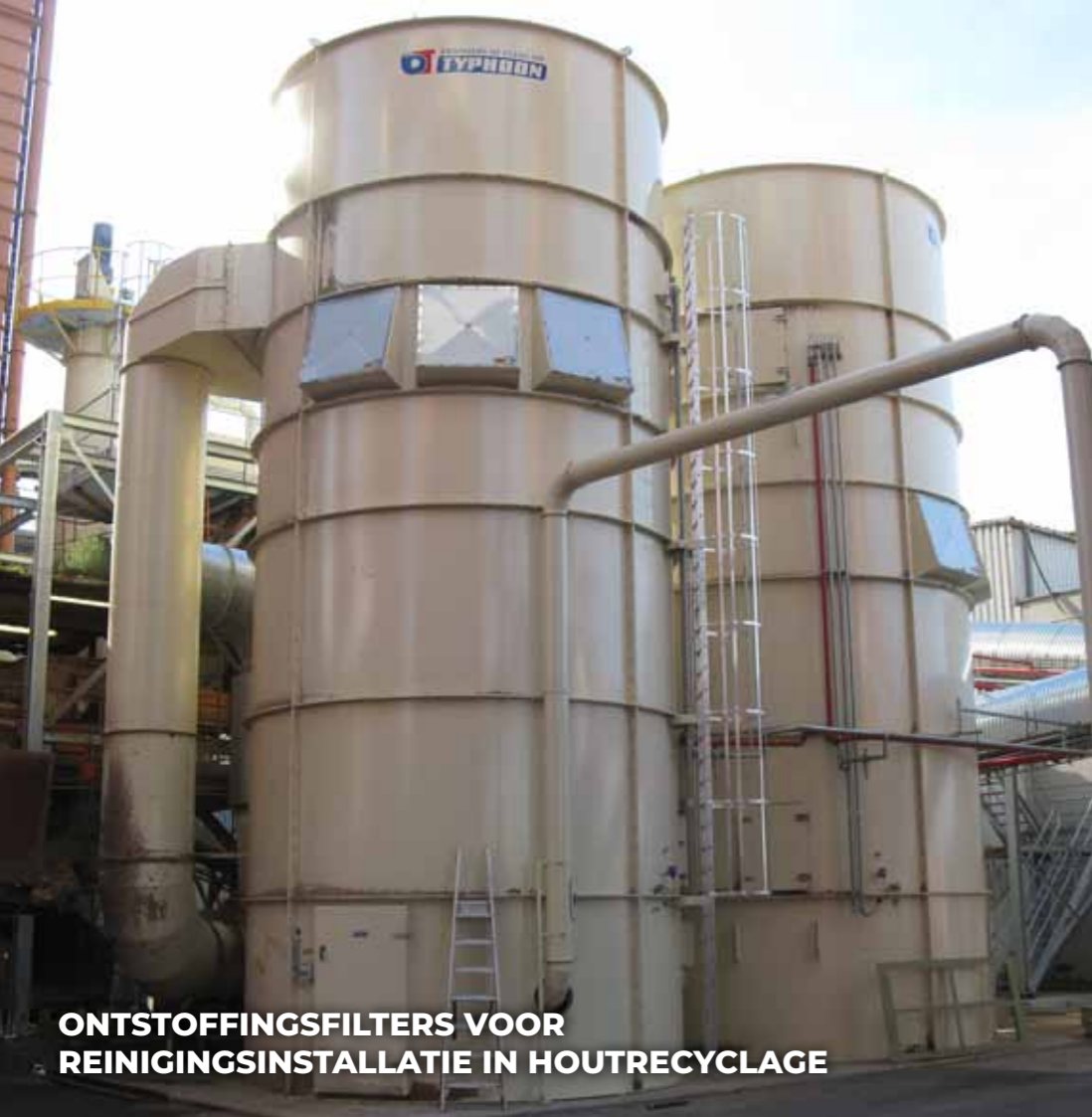
PNEUMATISCH TRANSPORT VAN HOUTSPANEN IN CYCLOFILTER
